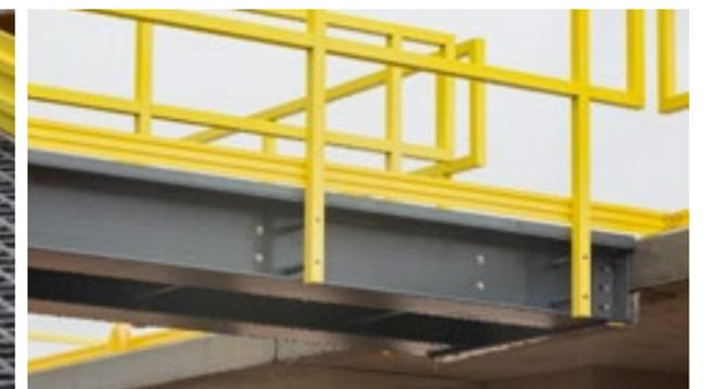
PROGrid® molded grating features a non-slip surface for a safer work environment. All of the handrails and stair towers were fabricated per OSHA regulations.
